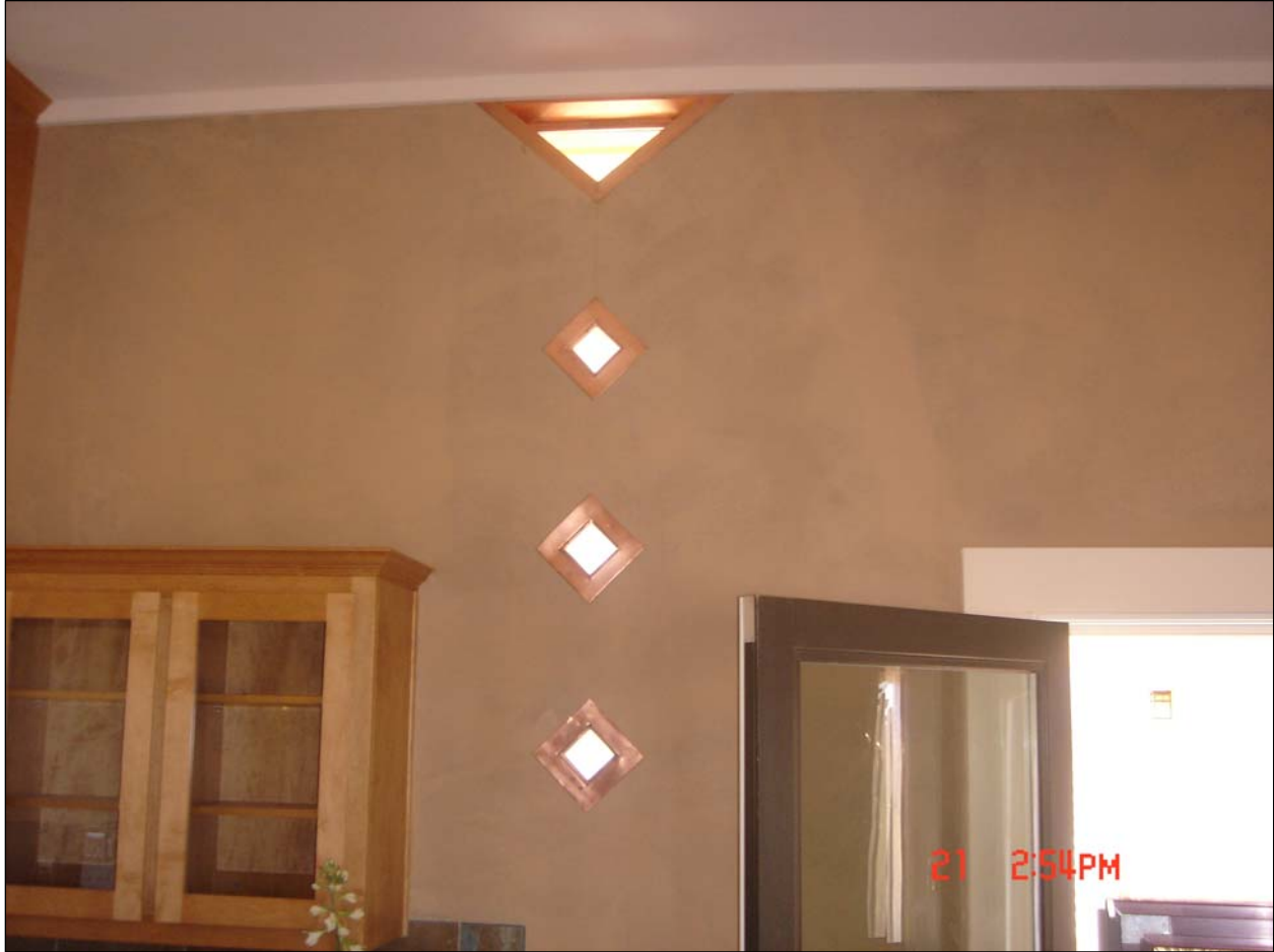
Figure 8: Custom Site Built Glazed Areas: Wall Penetrations
